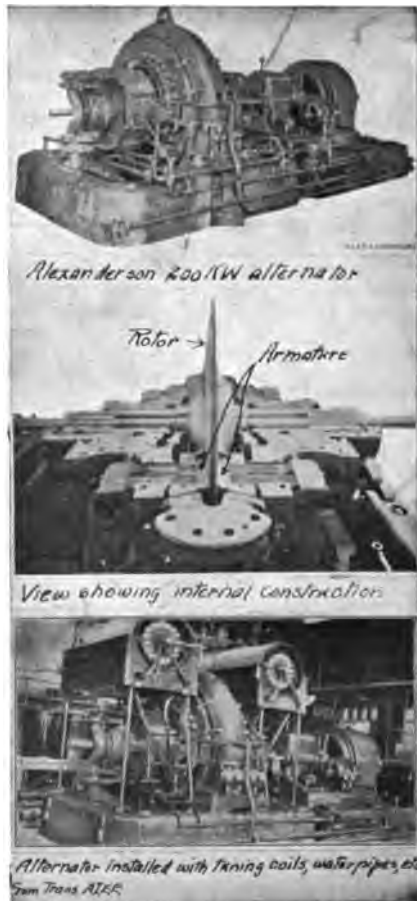
FIG. 17. Views of the high-powered Alexanderson generator installed at New Brunswick; over the alternator (in the lower view) may be seen the oscillation transformers which connect the generator to the antenna.
